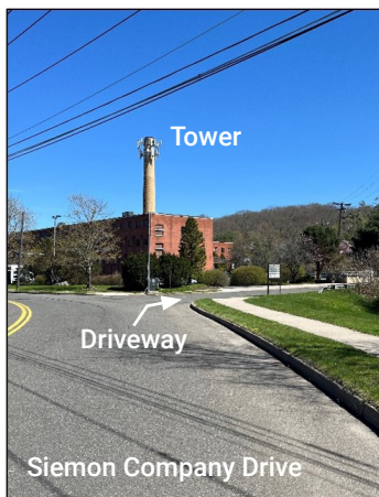
Driveway (From Siemon Company Drive)
